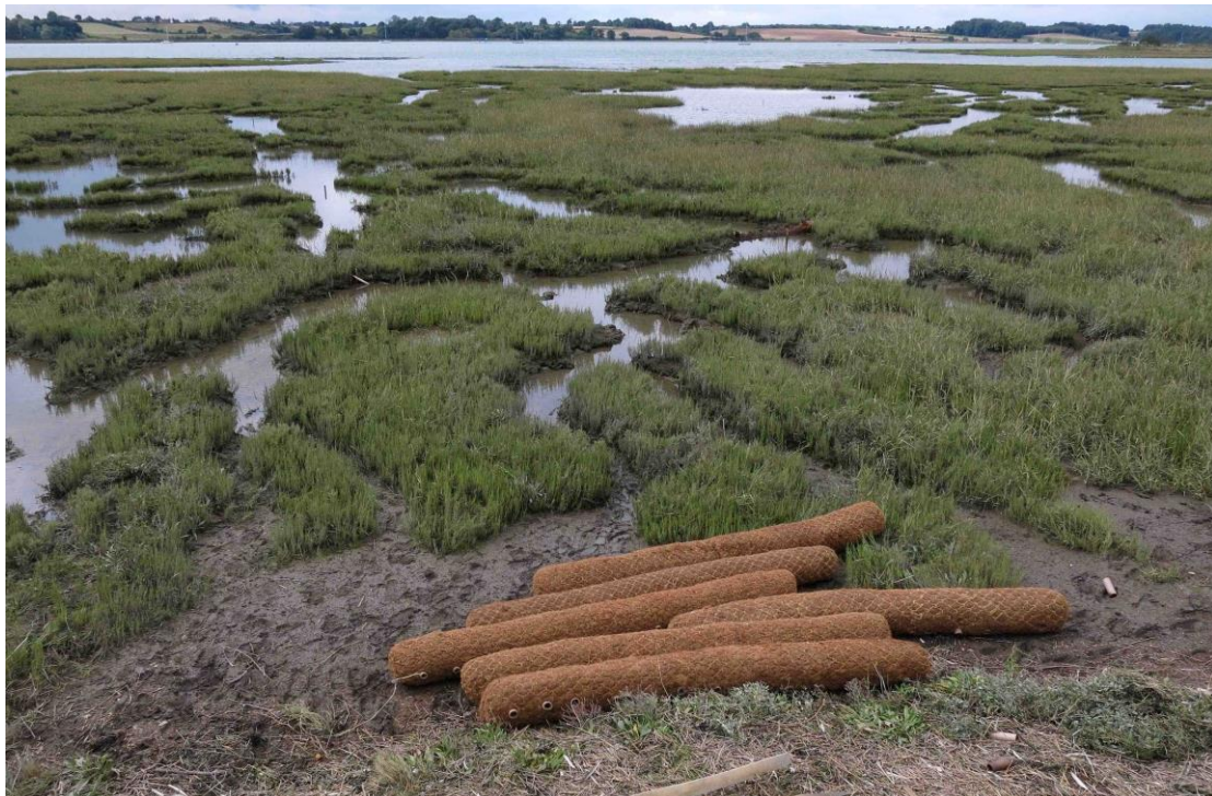
Coir Logs to be located in the channel system
