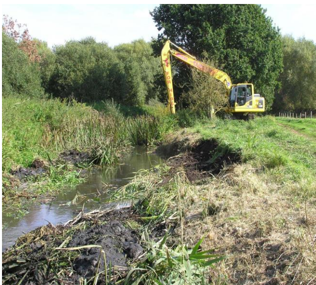
River channel restoration on the Little Ouse in 2013 reduced silt deposition by narrowing the channel to increase flow velocity
